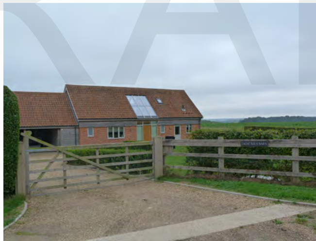
Timber cladding and glazing to a modern house near Holt
