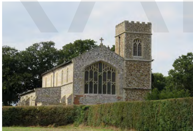
The rebuilt church at Edgefield
