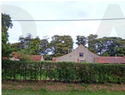
Converted farm buildings at Swan Lodge
