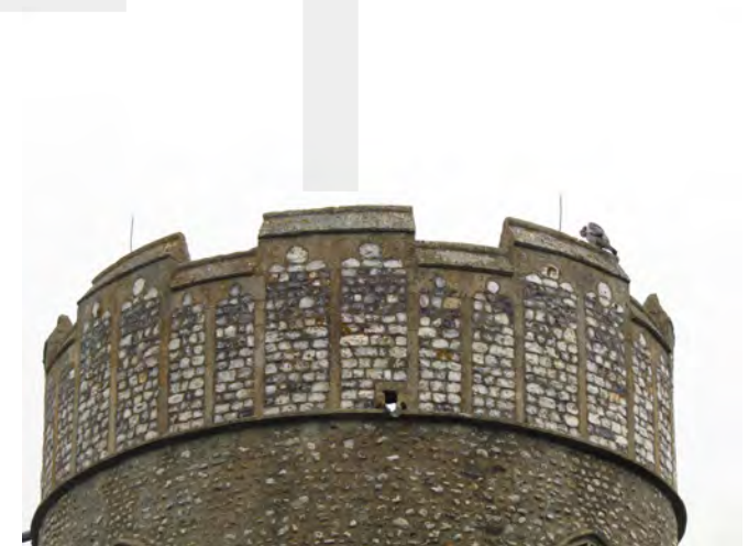
Knapped flint flushwork
