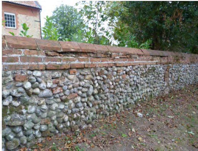
Flint and brick wall to The Mount near Edgefield
