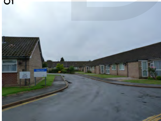
Late-twentieth century housing development on the northern outskirts of Holt
