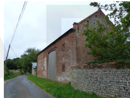
Converted threshing barn near Edgefield Old Rectory
