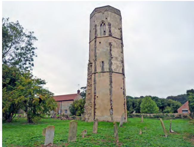
Stone used at the former Edgefield Church
