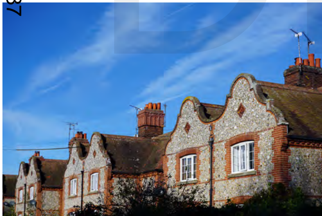
The cottages in Glandford have Dutch gables illustrating how the feature had become part of the character of the Glaven Valley
